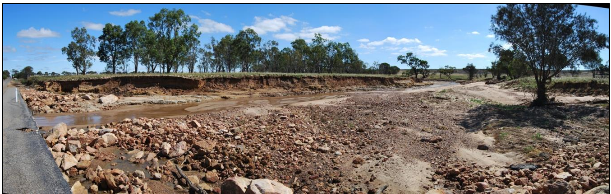
Jackitup Creek at Formby South Road crossing in March 2017 - looking downstream
