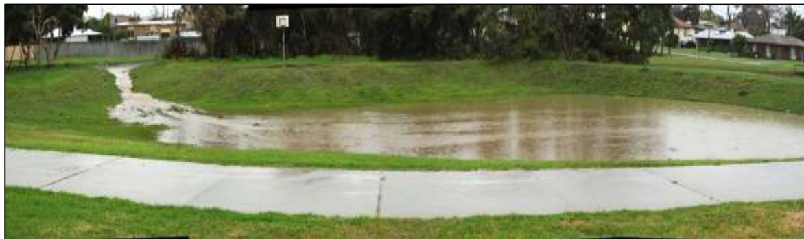
Figure 4: The detention basin at Dunn Park after receiving flow from a storm event. The initial flow enters the basin via the diversion channel at the left. A good quality patch of remnant vegetation (rare along Yakamia Creek) can be seen in the background.
