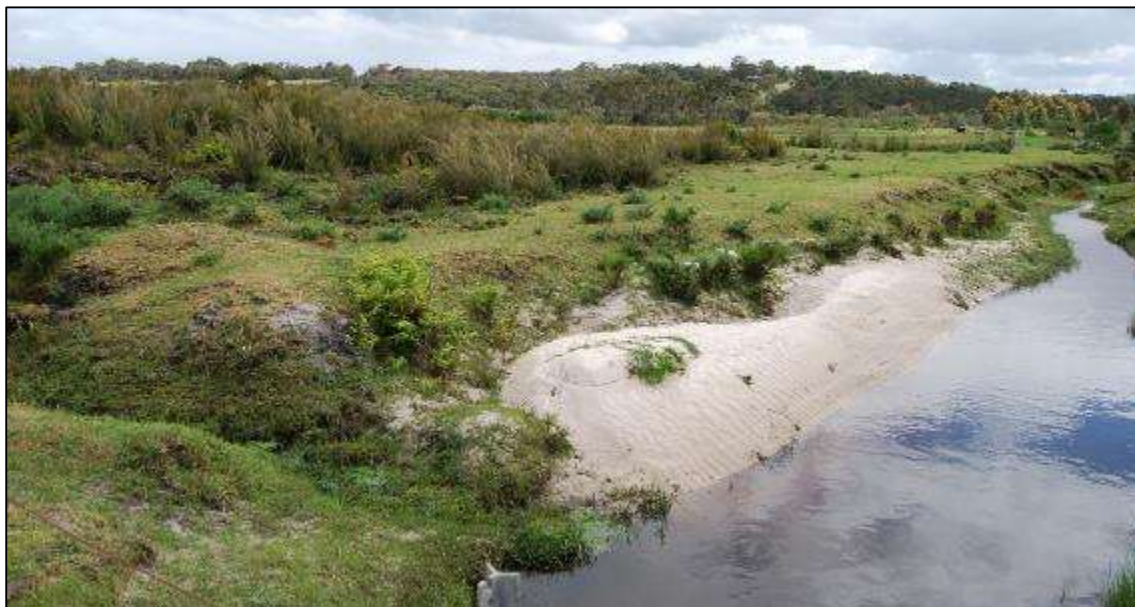
Figure 12: Sediment deposition in Yakamia Creek showing natural channel bank reconfiguration. Photo taken November 2014.
