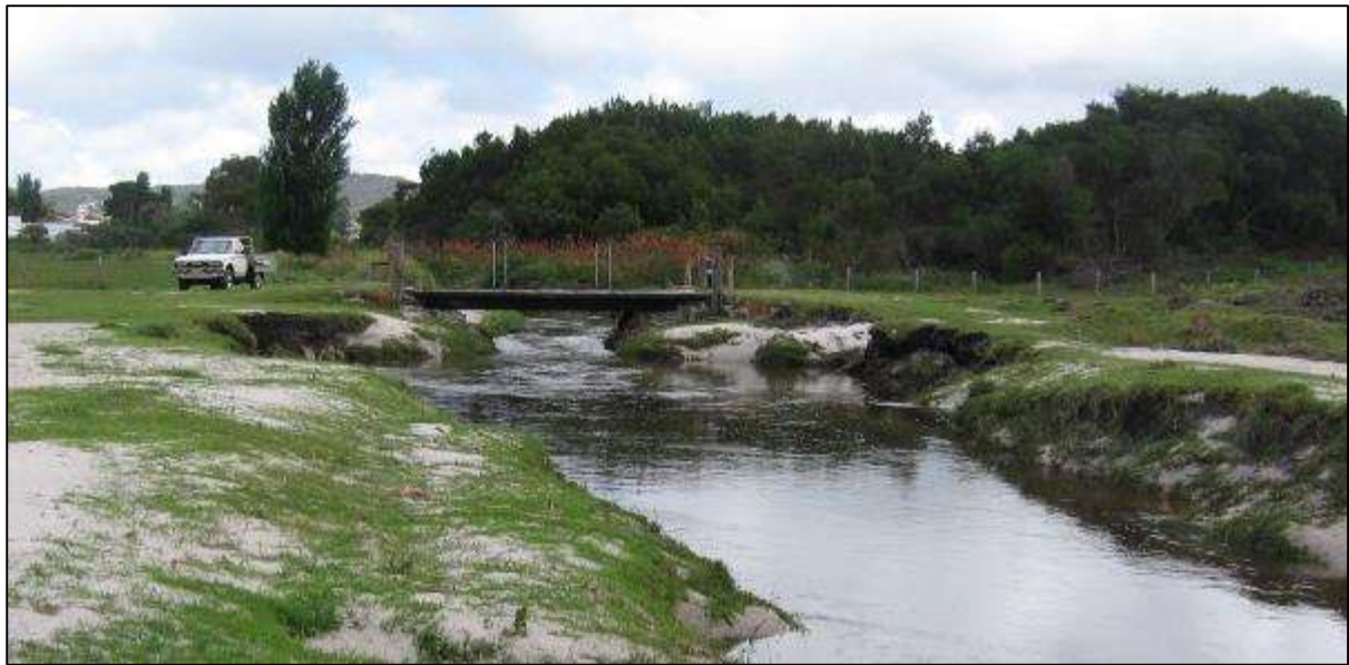
Figure 20: Yakamia Creek, looking upstream at the crossing and widened channel downstream created by turbulence. (2005 flood photo courtesy of Wilhelm Ficko).
