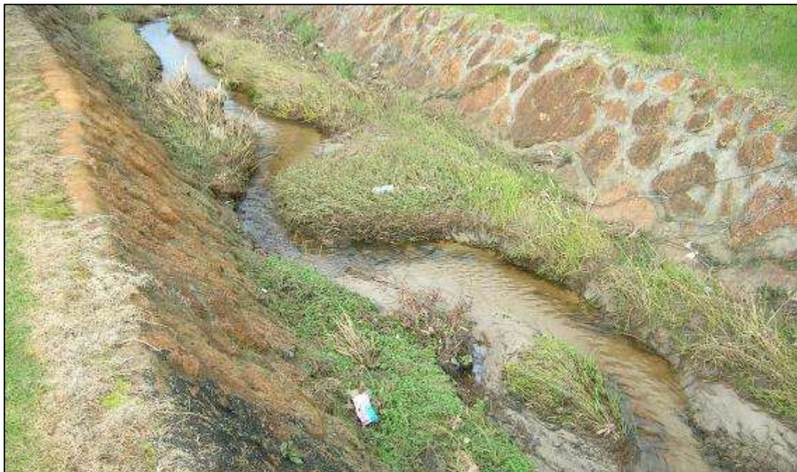
Figure 15: Armoured section of Yakamia channel upstream of the Aquatic Centre (2007).
