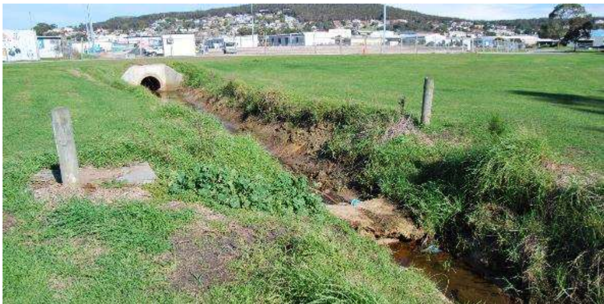
Figure 6: Drainage from Graham Street enters Yakamia Creek from behind the PCYC. There is opportunity to provide some bio-filtration function and improved visual amenity here.
