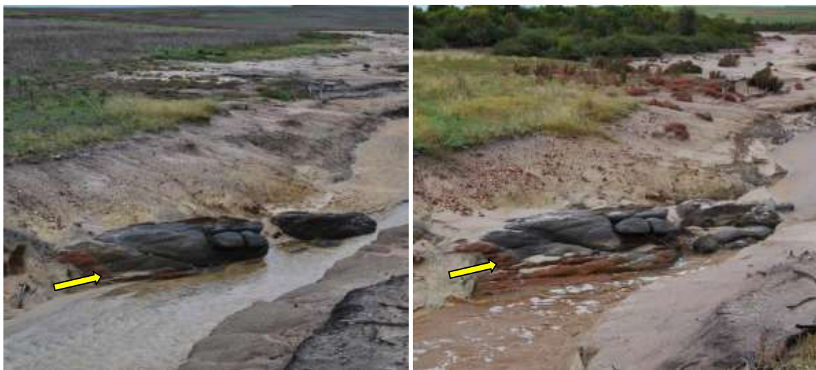
Figure 11: Photo point 06. 28 th February 2011 and 10 th June 2016. Note the channel deepening and exposure of more of the rock bar.
