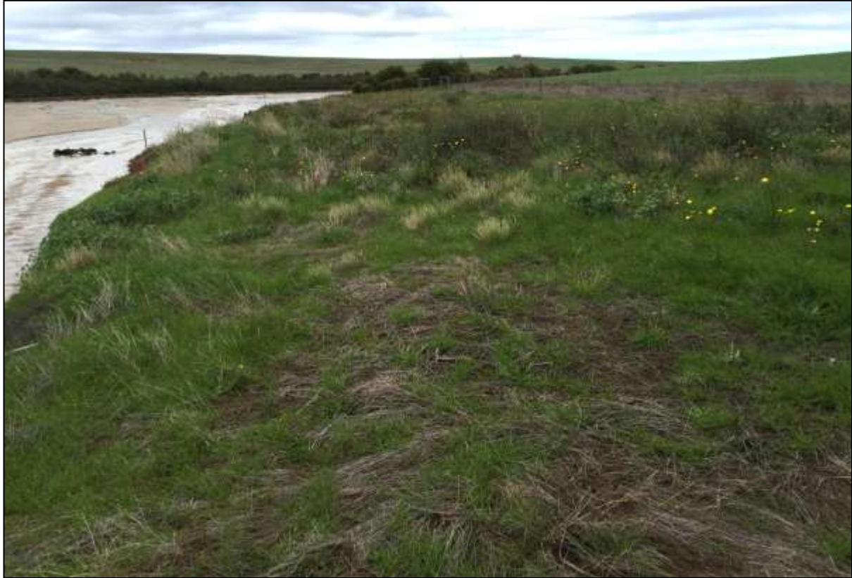
Figure 29: Un-revegetated section of the right hand bank.
