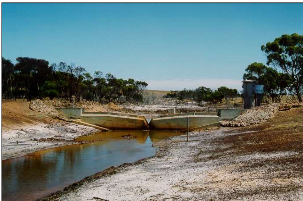
FIGURE 15: MELALEUKA GAUGING SITE. AT THE TIME THE PHOTOGRAPH WAS TAKEN THE STREAM WAS TRICKLING AND HAD A CONDUCTIVITY OF APPROXIMATELY 138 mS/cm (2.5 x SEAWATER). (PHOTO USED BY PERMISSION JANICKE DEPT OF WATER 2003)
