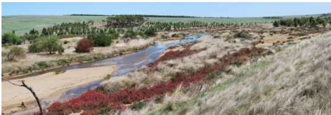
Restoration works on Yerritup Creek. Note the sediment plume moving down the creek-line.
