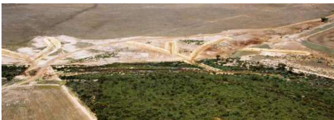
Drainage and access track compromising the connectivity of the riparian corridor in the middle reaches of the Lort River.
